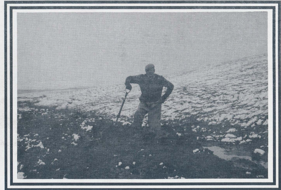
Jack, repairing Cam Fell.
