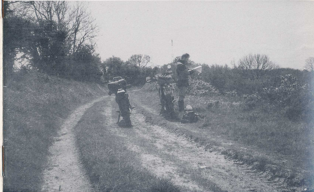
Old Furzey Road, ST 643 018. Picture by Dave Tilbury
