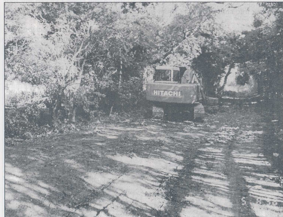
Photo by John Buswell - NCC Repairs Underway
