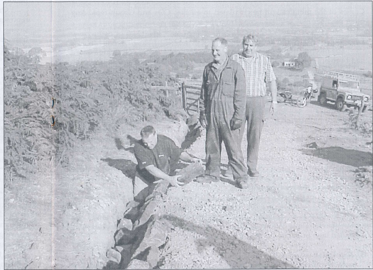
WEEKEND WORK: left, the state of the road before repairs started, and right, gullies are lined with sandstone by the TRF volunteers.
